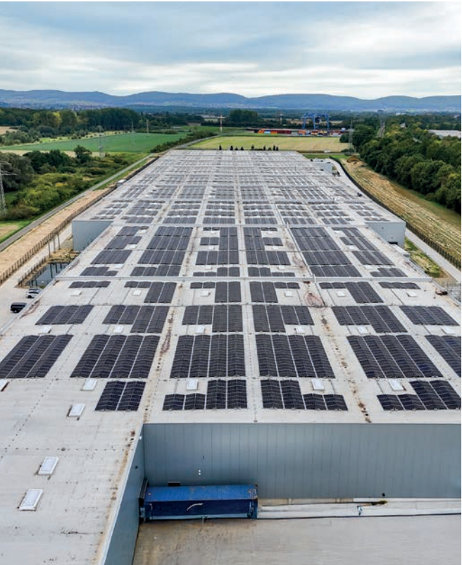
We also live sustainable logistics in contract logistics, as this flagship project at RegioPort Minden demonstrates.
